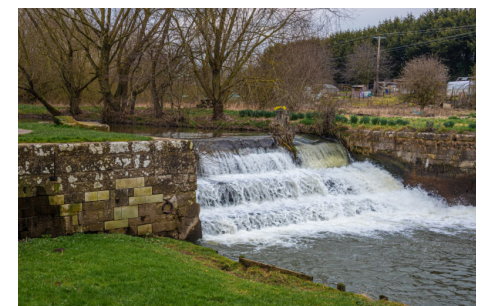
HARBOUR WALLS AND WEIR - BEDALE
